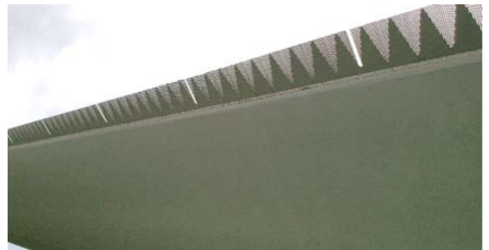
Figure 4. Applying metamaterial on the fan housing for LFN mitigation [17]
